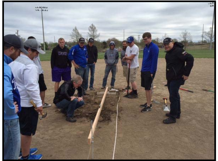
Turf students at K-State show how to build a mound by Dale Getz and Boyd Montgomery of The Toro Company.
