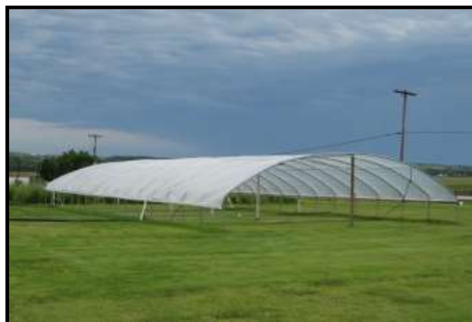
Figure 1. Stationary rainout shelter.
